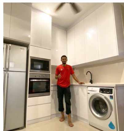
Final installation of kitchen cabinet
